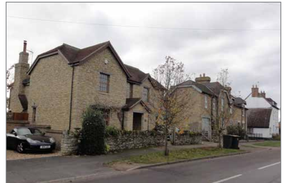
Fig. 5.2.4 Local example of representative building typology.
