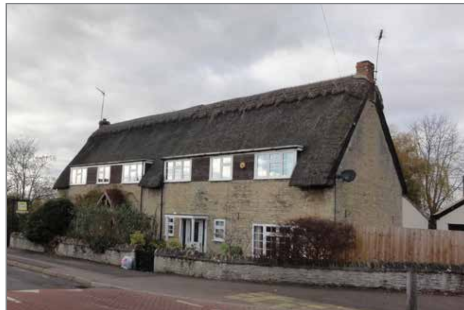
Fig. 5.2.2 Local example of representative building typology.
