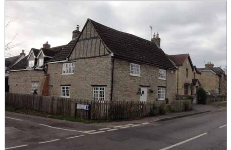
Fig. 5.2.3 Local example of representative building typology.
