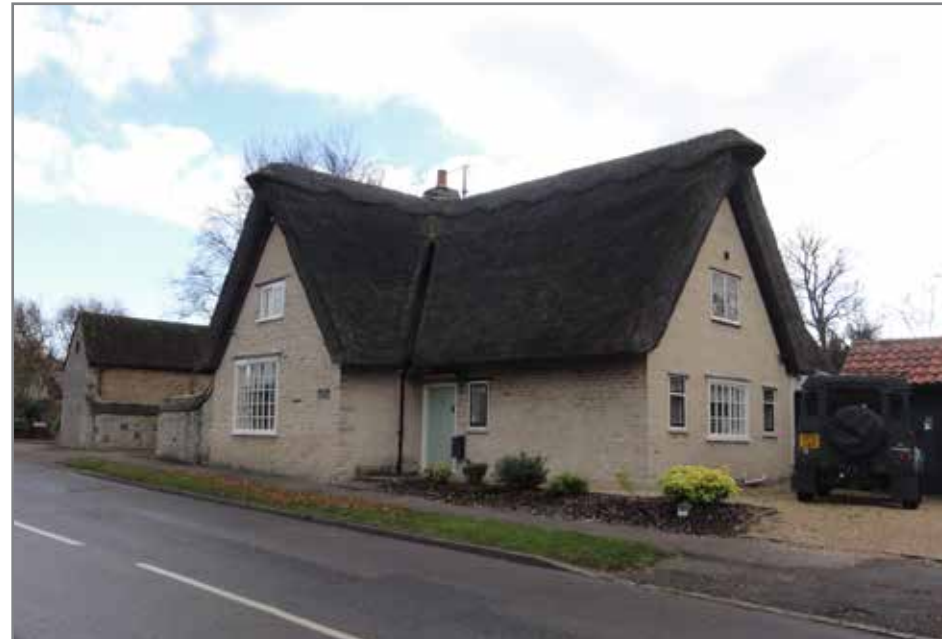
Fig. 5.2.1 Local example of representative building typology.
