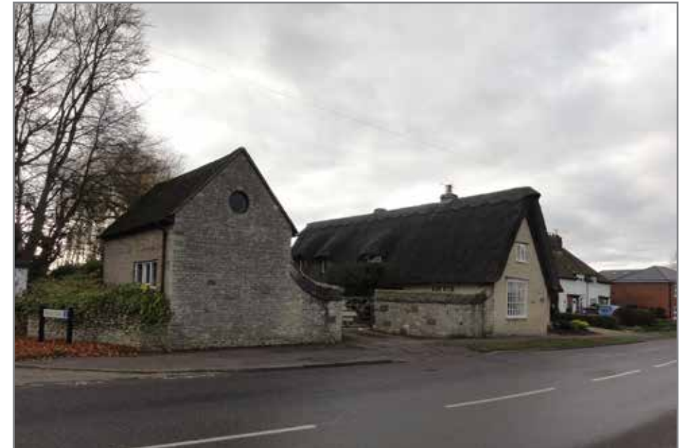
Fig. 1.4 Listed building on Radwell Road
