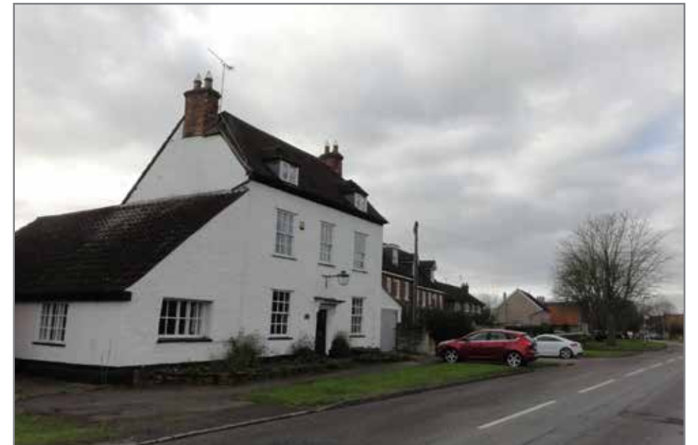
Fig. 1.5 Listed building on Radwell Road
