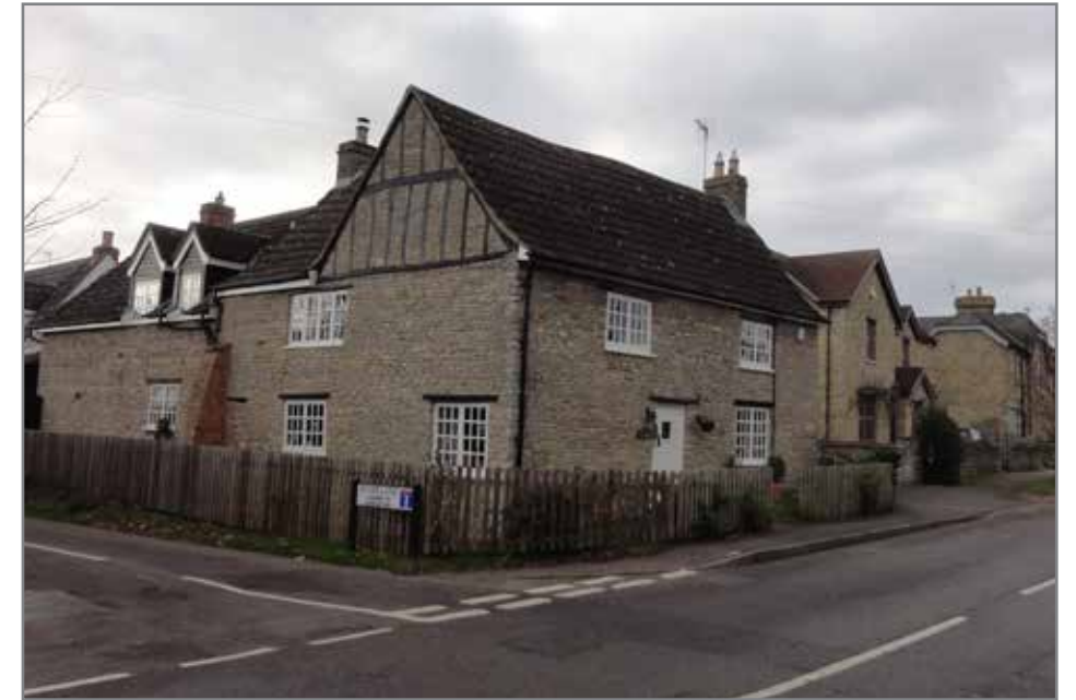
Fig. 5.2.3 Local example of representative building typology.
